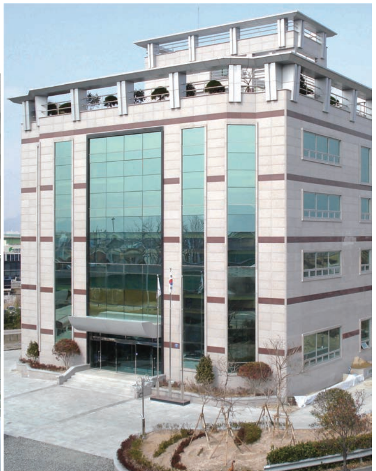
Chosuk C&D office building
