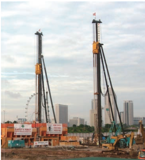
Marina Coastal Expressway C487
